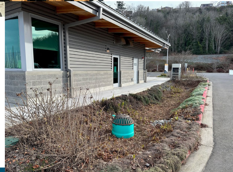
Bioretention at Shilshole Bay Marina
