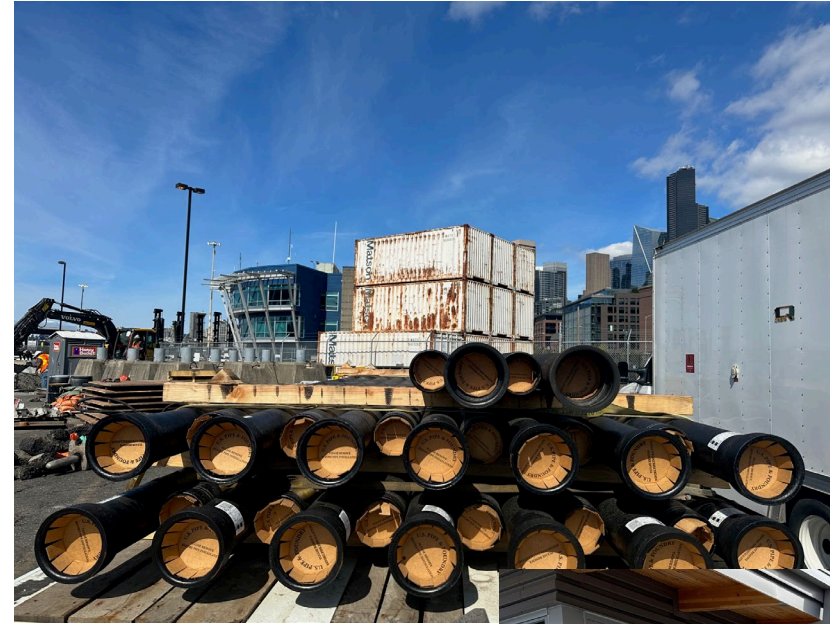
Pipes ready for installation at Terminal 46
